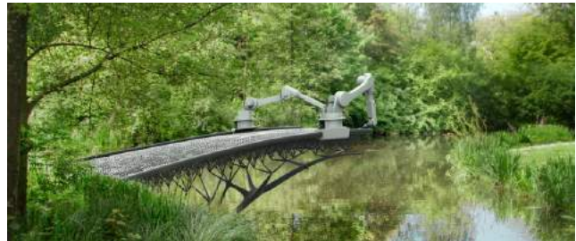
Fig. 9 A bridge to be fabricated by a robotic platform. The bridge under construction shall support the movable robotic platform at all intermediate stages. Image courtesy of MX3D ( www.mx3d.com ).
